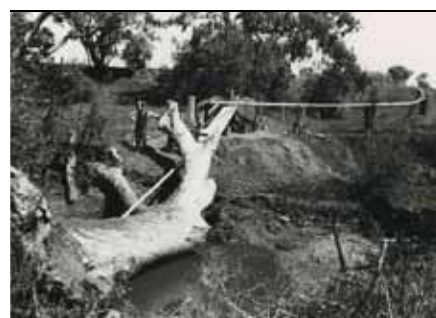
Figure 3.19 Charles Cobb Ragless pumping water from Wattiparinga Creek to irrigate the vineyard on Tonsley (Section 63) in 1935. The pump was driven by a McCormack-Deering Tractor. Photo courtesy of the State Library of South Australia, image B 33775.
