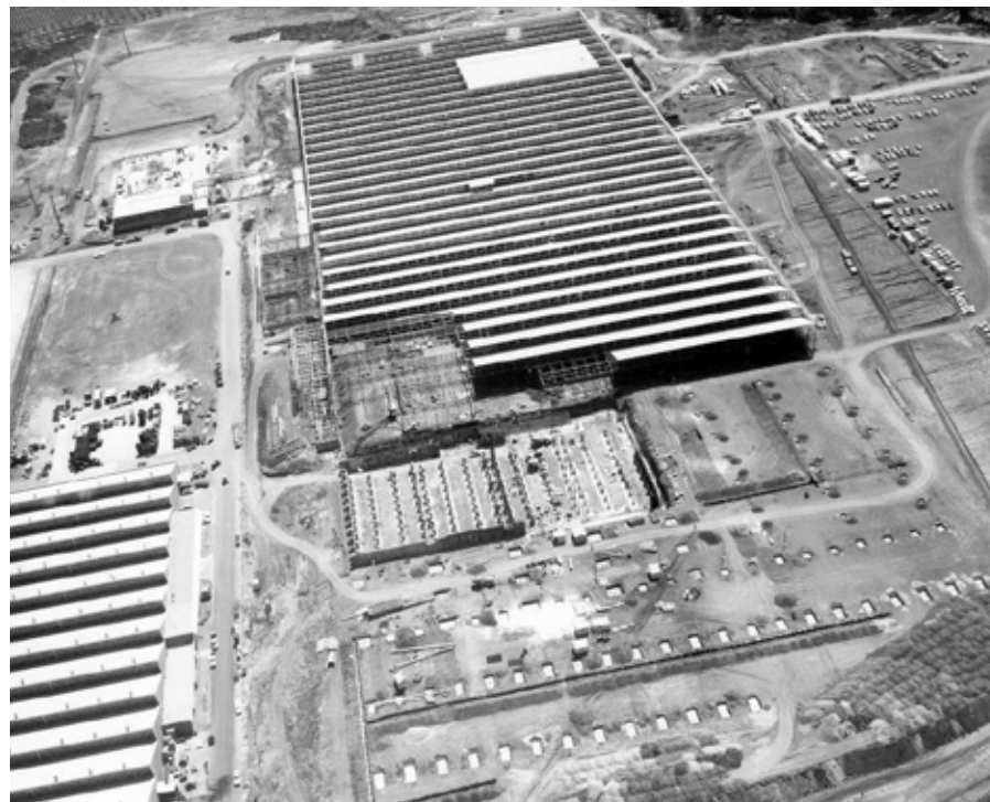
Figure 3.35 The main assembly plant at Chrysler in April 1964. Source: DMITRE/MMAL.
